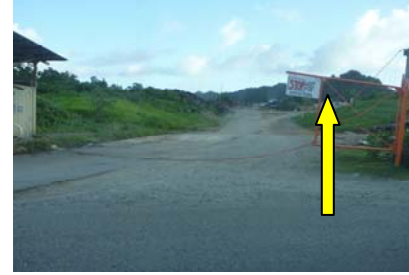
Unsecured Gate and Waste used as Slope Formation
